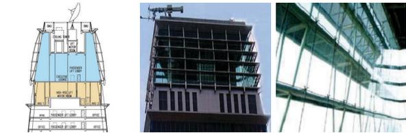
17m 높이의 Pent House Pin Fixing Frameless Glass Wall
